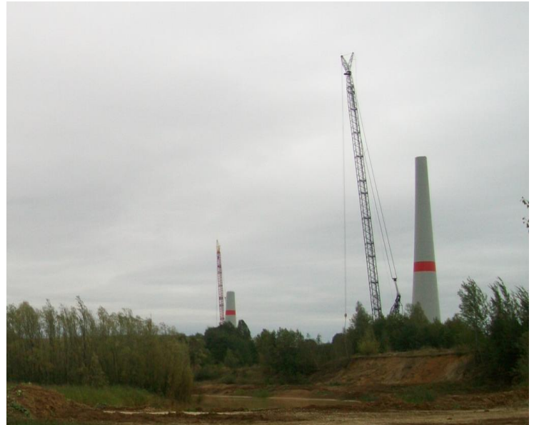
Wind Works Project Burg 2 while in construction in 2013
