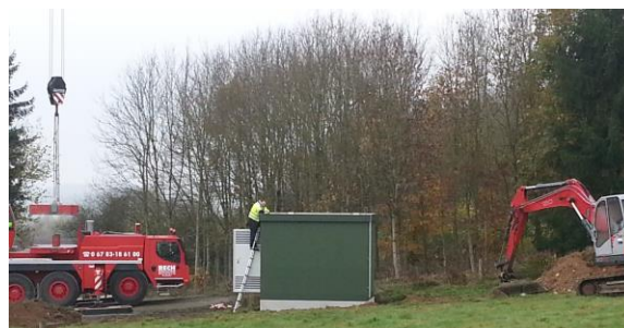
Work at Wind Works interconnection station
